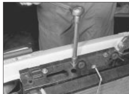
3.4a Undoing radiator retaining bolts
